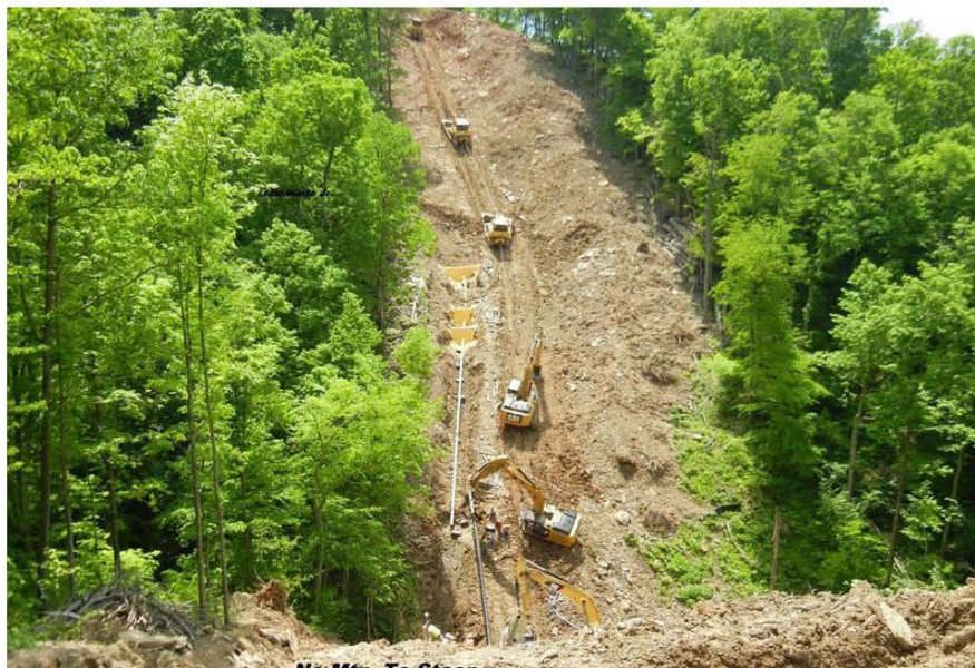
Because there has been no construction on the proposed Dominion pipeline, this picture could not possibly show disturbance in the Monongahela National Forest. It is from somewhere in Wetzel County and demonstrates the perils of construction on steep slopes. Photo courtesy of Ed Wade.
